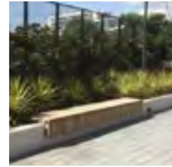
Concrete bench with timber battens
