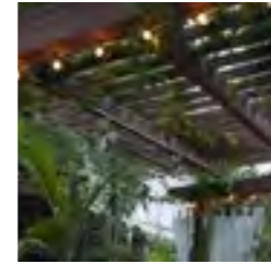
Timber pergola with greening
