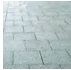
Concrete unit paving
